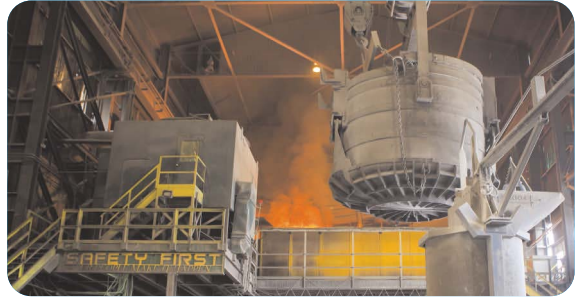
Nucor Steel optimized its steel melting process to drastically reduce electricity consumption.
